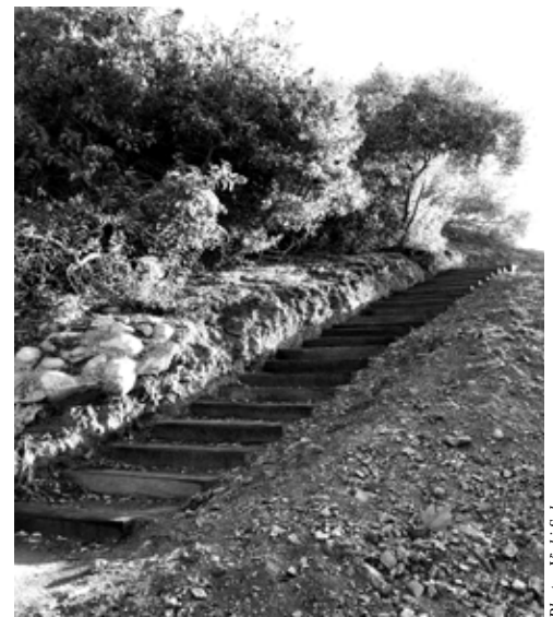
New stairs at Sycamore Canyon.
